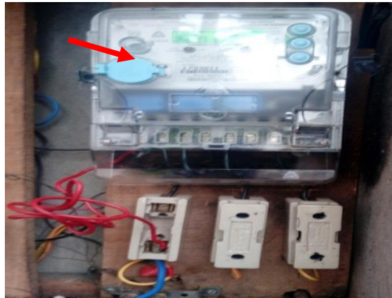
Fig.7. Direct Tapping in Three Phase Meter
